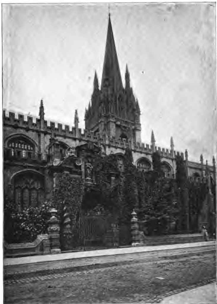
ST. MARY'S, OXFORD. TOWER PARTLY CONTEMPORANEOUS WITH WYCLIF.
