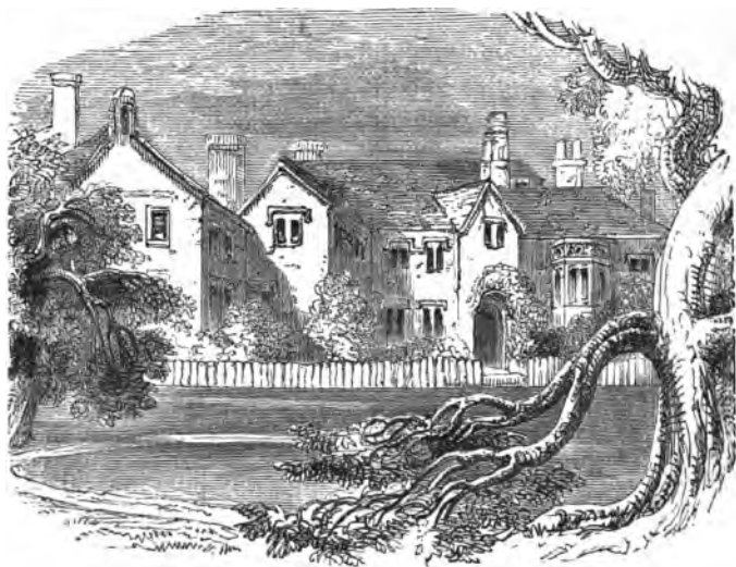
MANOR HOUSE, LITTLE SODBURY.
